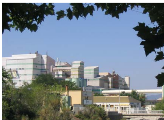
Figure 1. Axens Salindres Manufacturing Site
